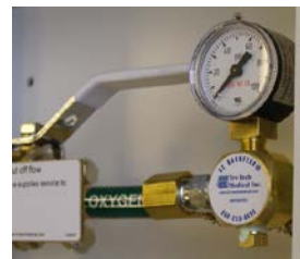
Single port E Z Backfeed™ fitting with Gauge & DISS gas specific demand valve on the right side port shown above
