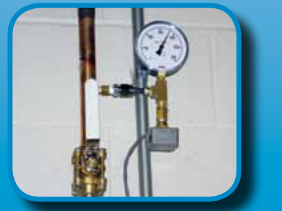
Genesys® PST assembly installed patient side of source valve
