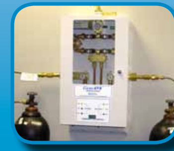
Models TMCU & TMLU fully automatic analog manifolds
